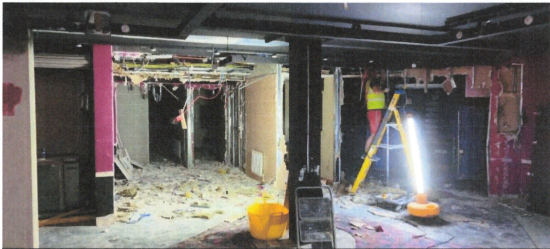
Opening up during construction
